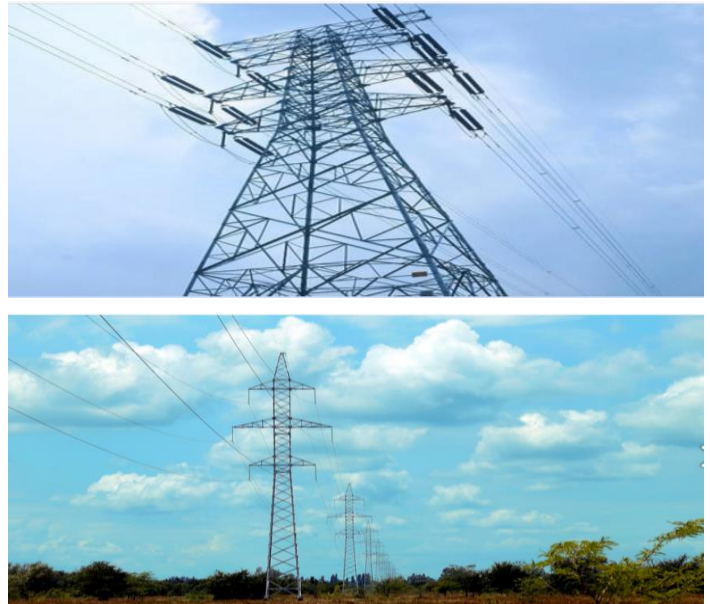
Figure 2. 220kV Double circuit transmission tower and line [33,34]
